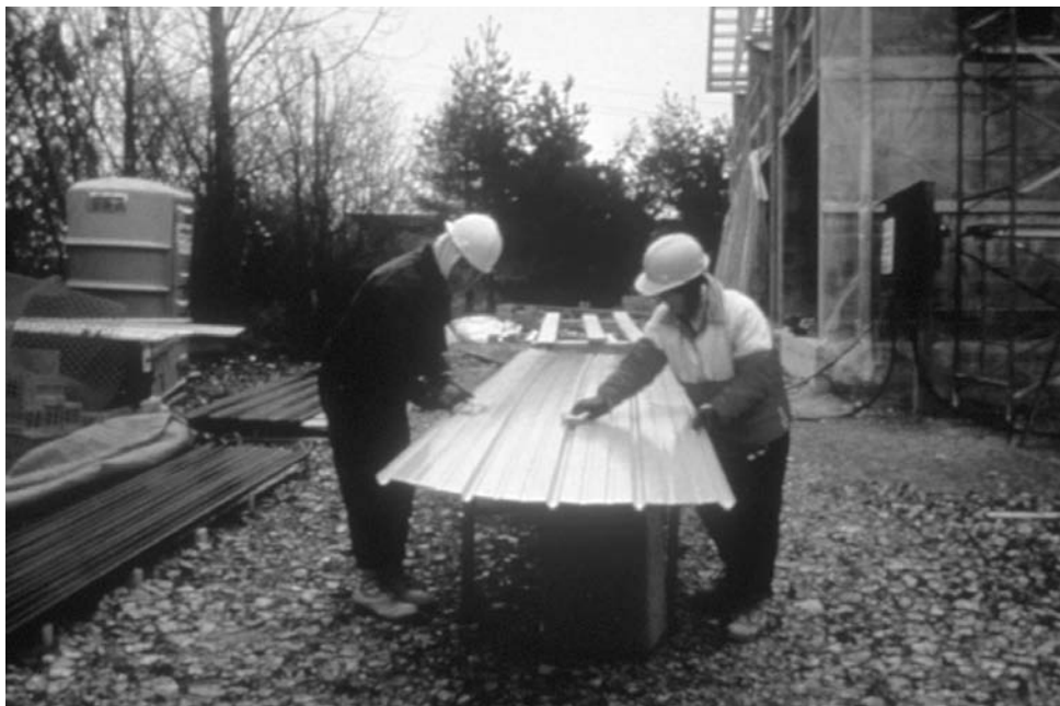
7.5 Barrhaven roofing being cleaned before installation.
