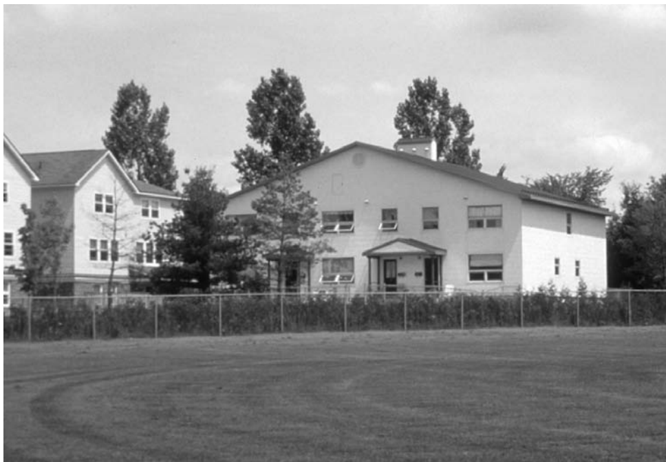
7.4 Barrhaven Community Housing for the Environmentally Hypersensitive. Exterior view across the 'pesticide free' municipal park.
