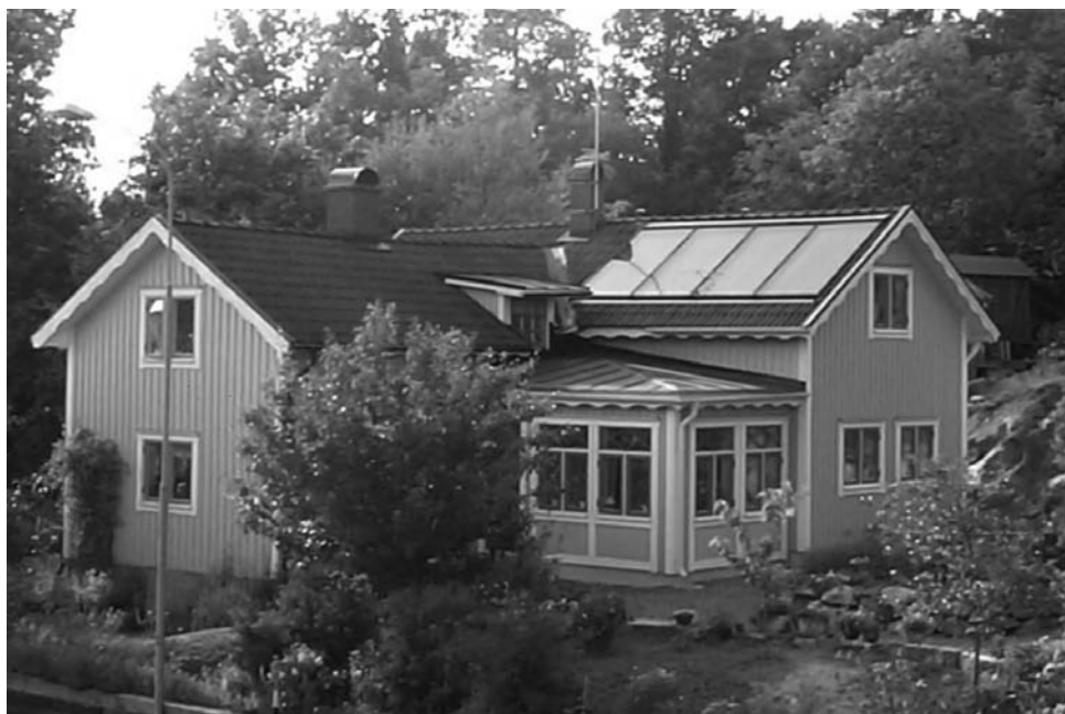
6.4 A solar collector on a typical single-family Swedish house.
