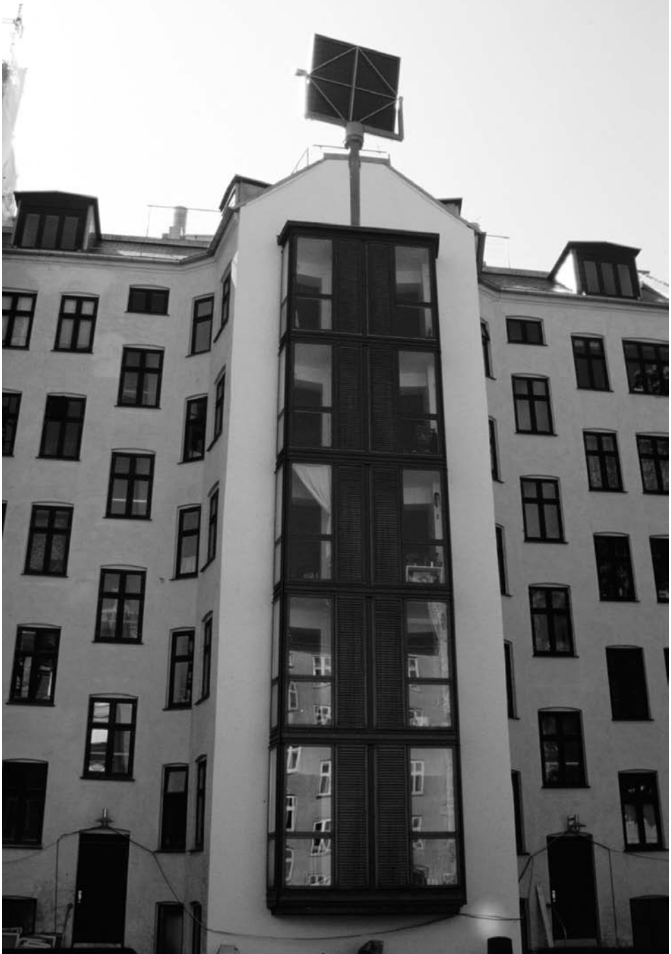
10.4 The Hedebygade project served as the Danish Ministry of Housing's 'flagship project' on urban ecology. On top of the building is a prism to channel daylight into the flats.
