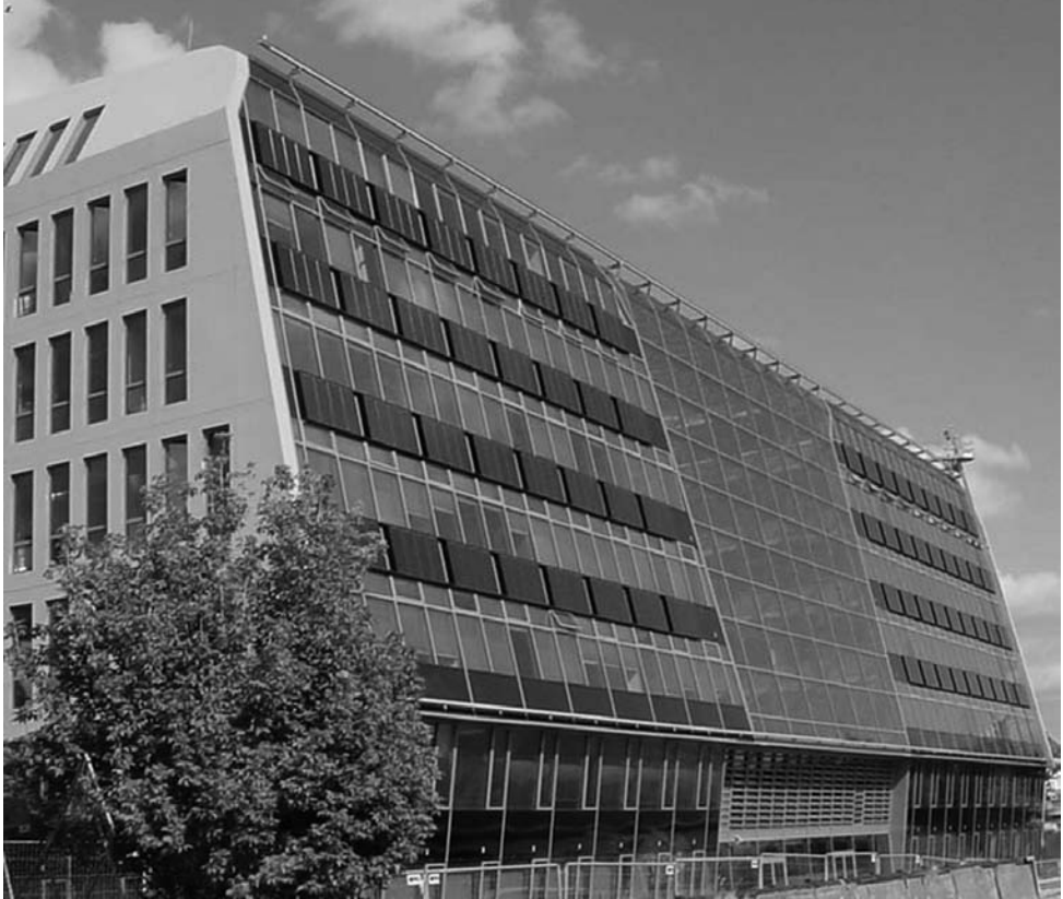
5.3 Photovoltaic panels integrated in the design of a Berlin office block.
