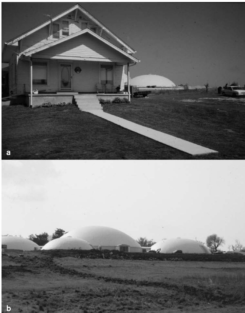
11.4a and b Two views of the domed school in the new town of Pattonsburg.
