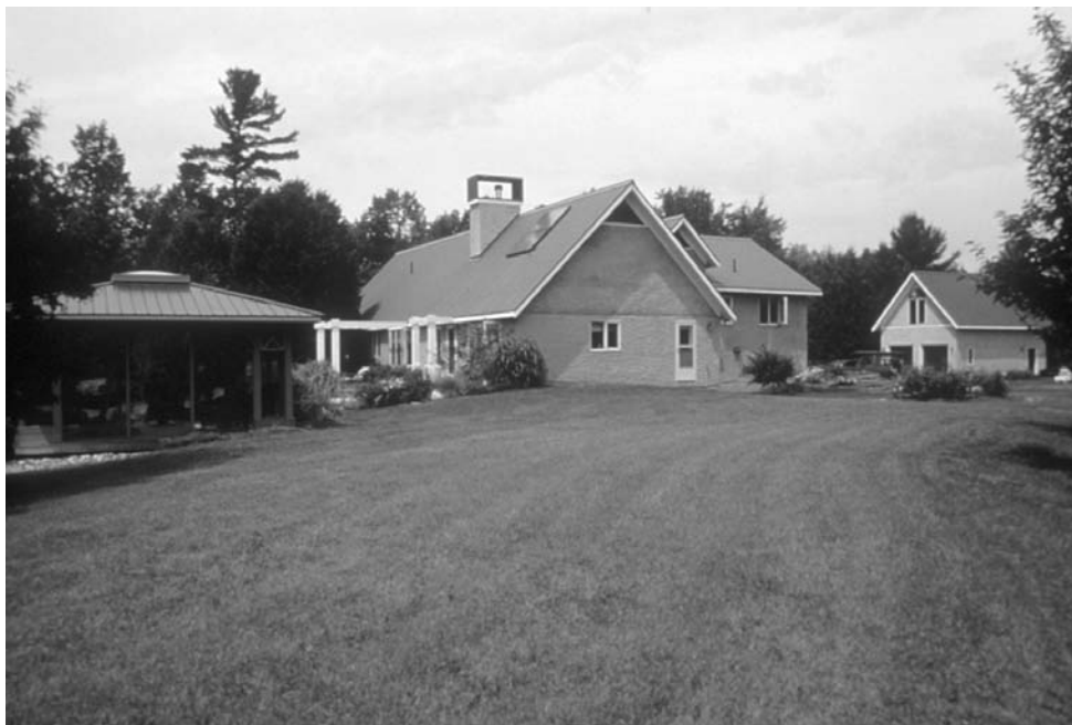
7.6 Exterior of the Nelms house.
