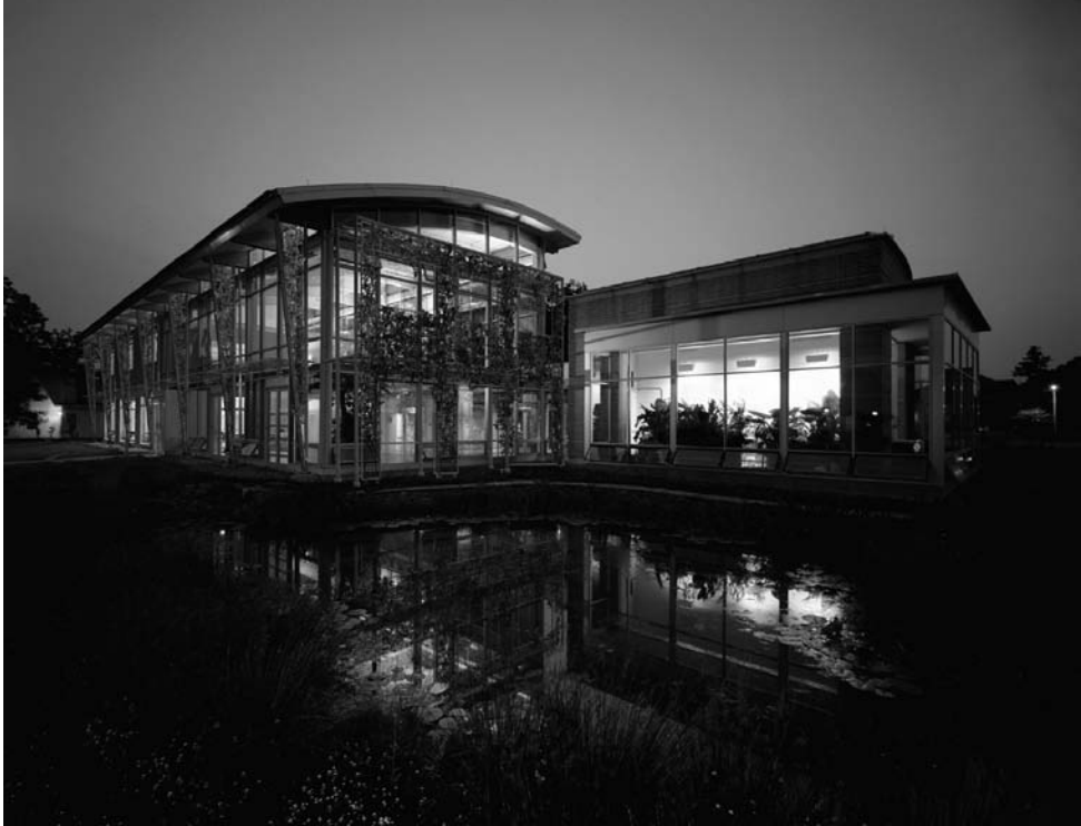
3.3 The Adam Joseph Lewis Center with south and east trellis.
