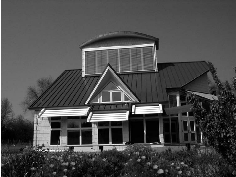
3.1 The Environmental Technology Center at Sonoma State University, California.
