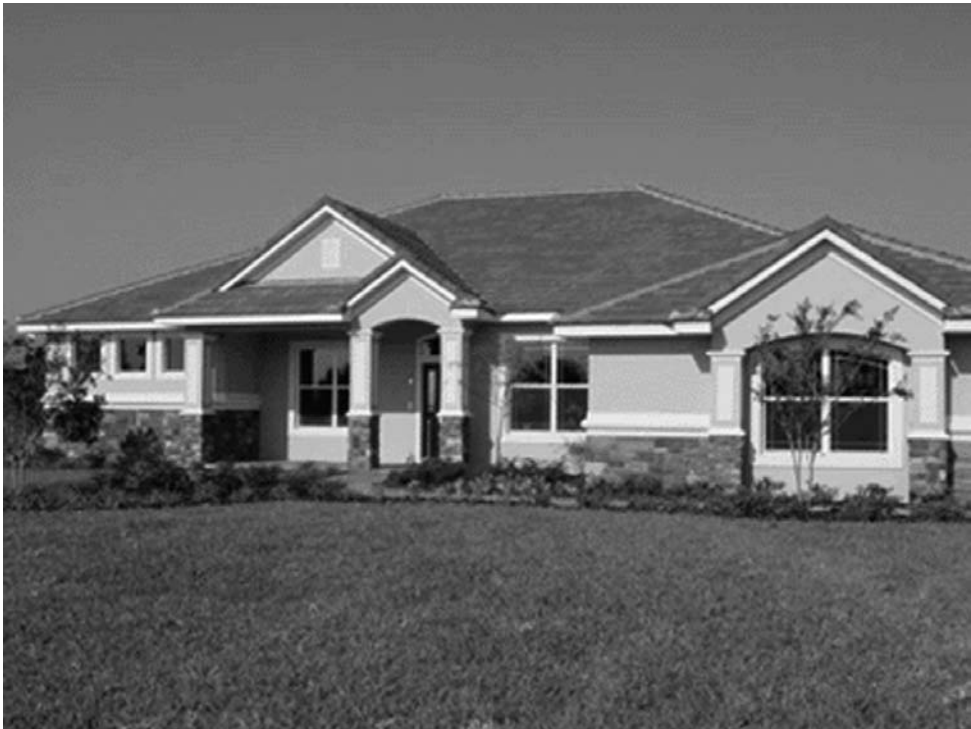
4.6 The first home rated under the Florida Green Building Coalition's Green Home Standard.
